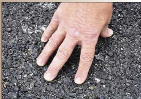
Porous pavement looks like regular asphalt without the tiny rocks.
