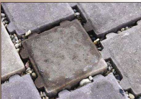
Modular pavers allow rainwater to go between the cracks instead of running into the storm sewer.
